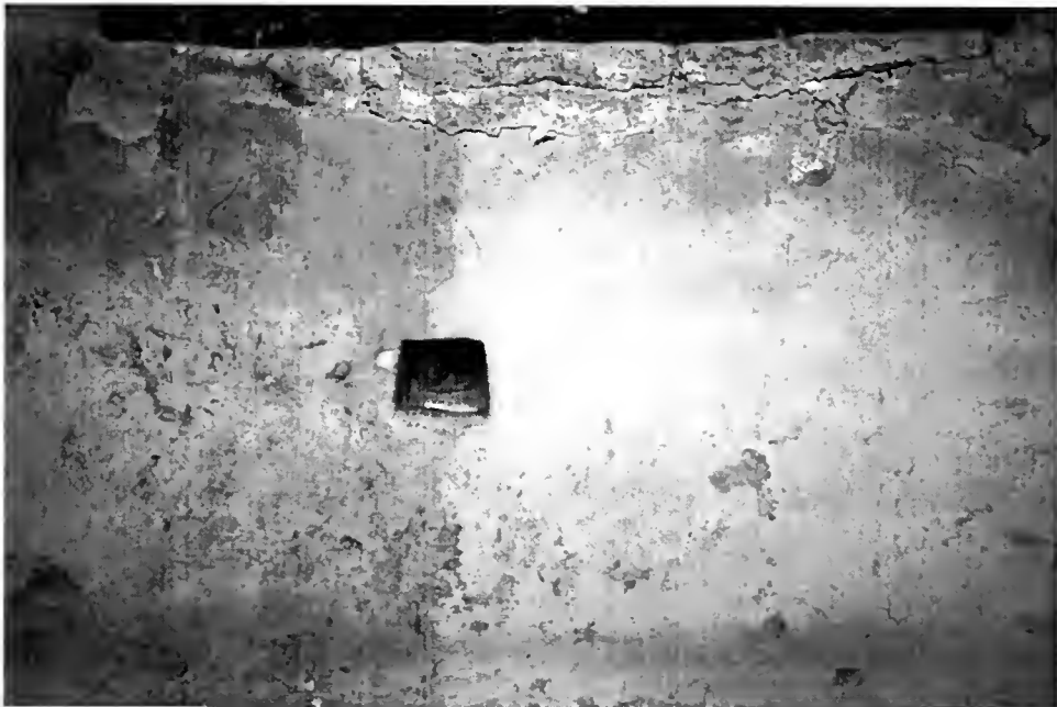
Figure 15. Kiva Q, dividing line in the uppermost finish layer.
